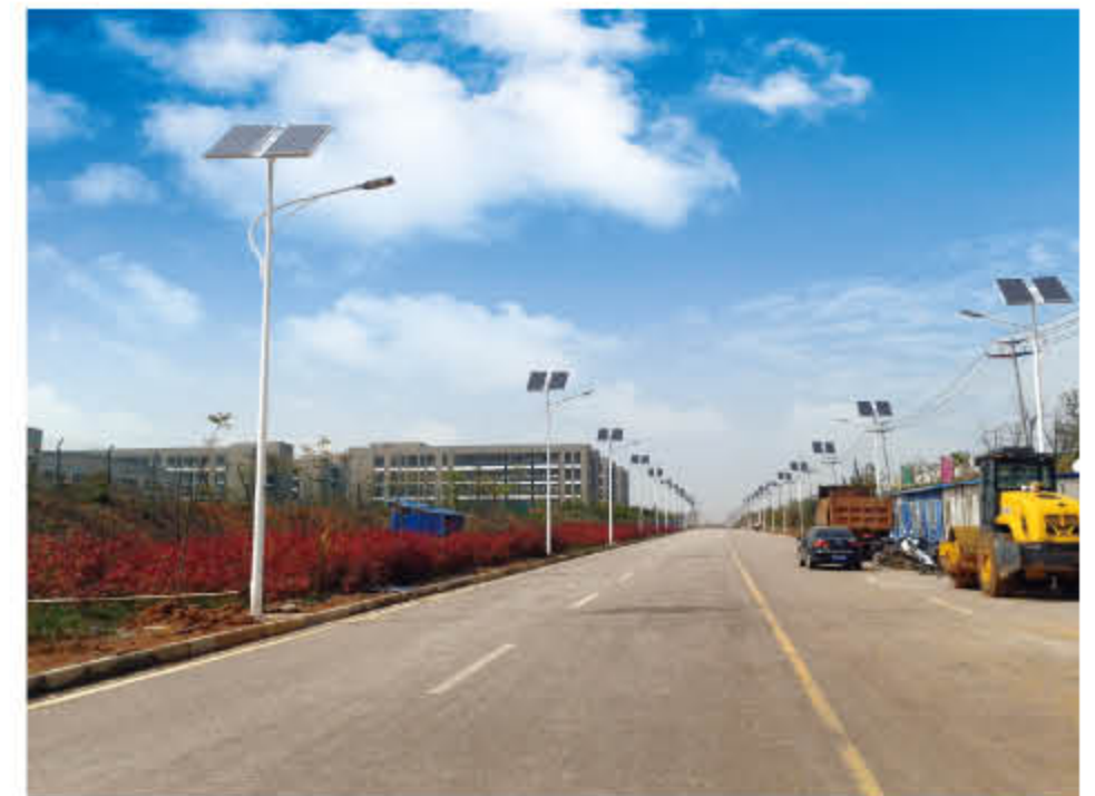
Anhui Wuhu Economic Development Zone, the Longitude 4th Road
